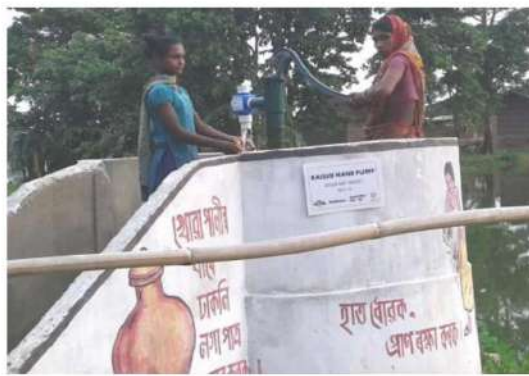
Hand pump fitted with PurAll –online chlorination.
